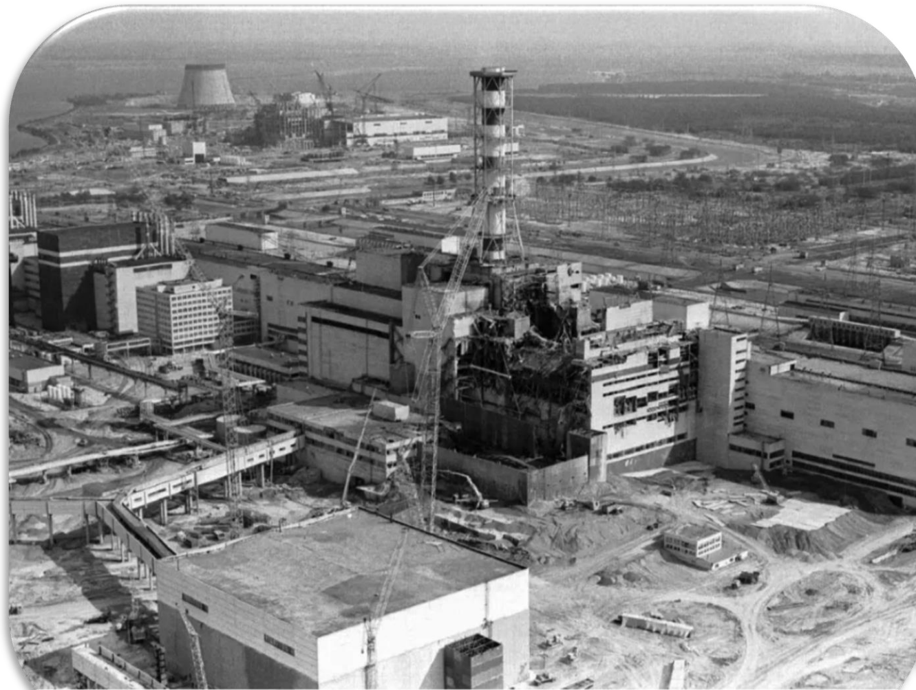
1986 aerial view of the Chernobyl nuclear plant in Chernobyl, Ukraine, shows damage from an explosion and fire in reactor 4 that sent large amounts of radioactive material into the atmosphere. Volodymyr Repik/AP
